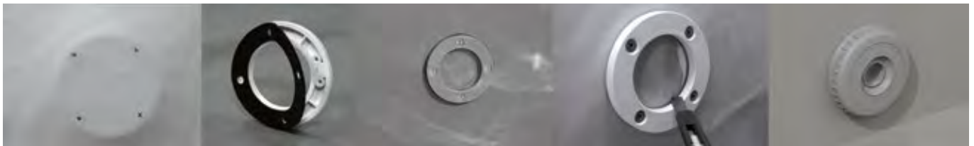
Figure 35 – Installing the return fitting flange
