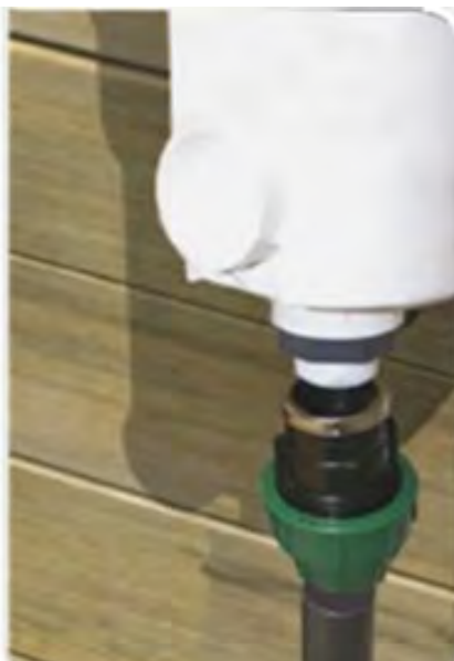
Rigid descending pipe under the skimmer
