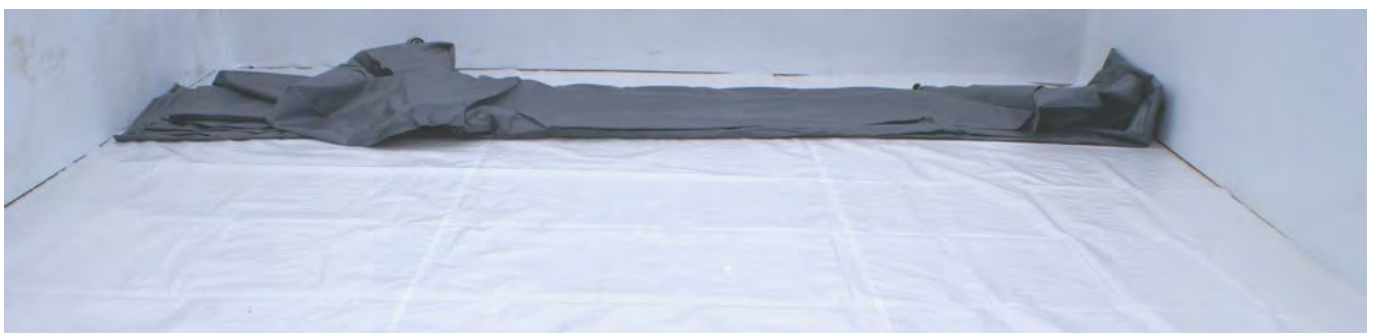
Figure 33 – Unfolding the liner
