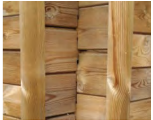
Figure 61 – Slotting together of the wooden slats
